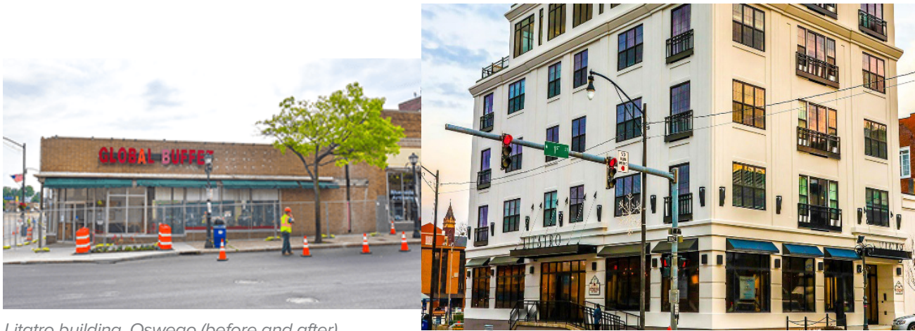
Litatro building, Oswego (before and after)
